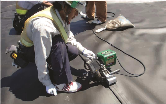
Self-propelled fusion Cross section of junction
