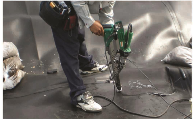
Extrusion welding Cross section of junction
