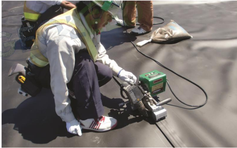
Self-propelled fusion Cross section of junction
