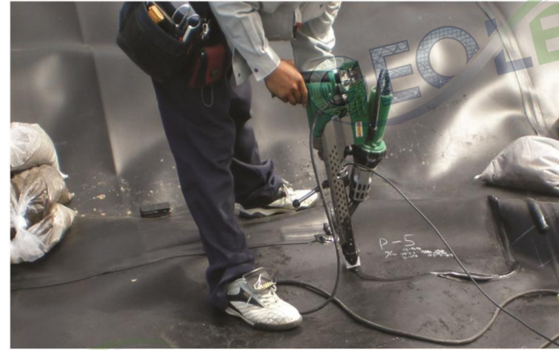
Extrusion welding Cross section of junction
