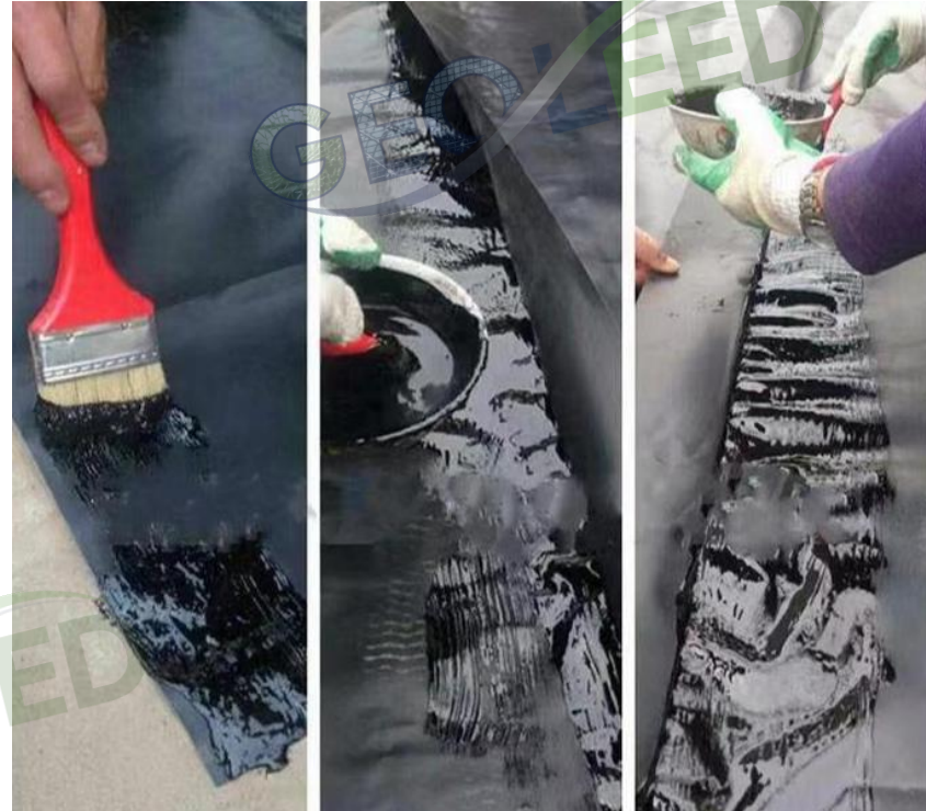
Adhesive bonding, joint width 50mm.
